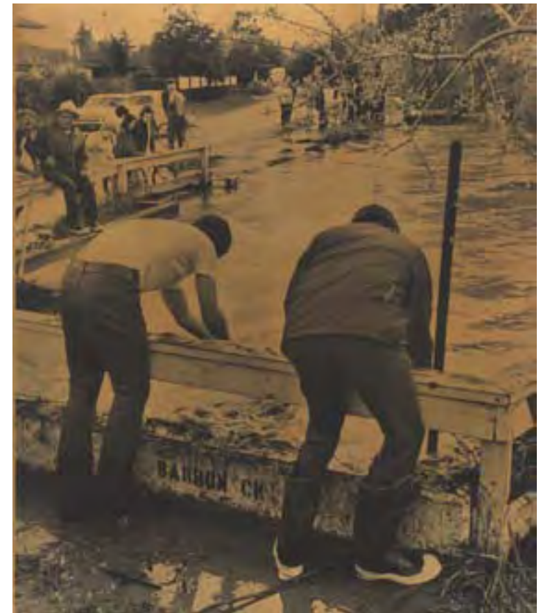
Volunteers clearing trash rack at Laguna Avenue culvert on Barron Creek during the 1973 flood. (PAHA Guy Miller Archives)
