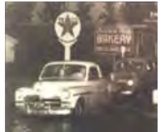
Overflow flooding on El Camino Real from Barron Creek, 1955. (Courtesy of the Santa Clara Water District.)
