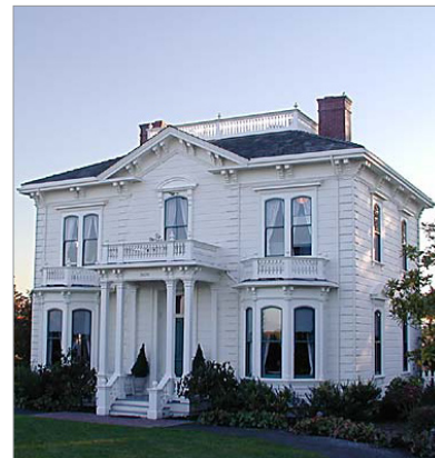
Historic Rengstorff House, conveniently located in Shoreline Park. (Courtesy of Friends of Rengstorff House.)
